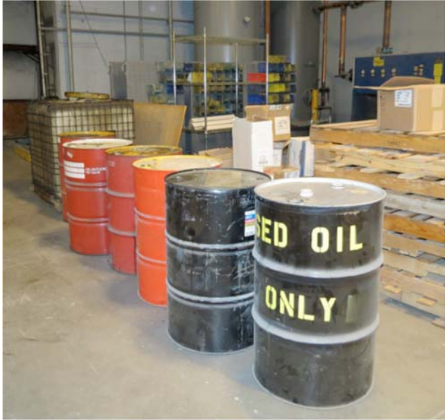
FIG. X1.1 Indoor chemical and used oil storage in 55-gal (208-L) steel drums.
