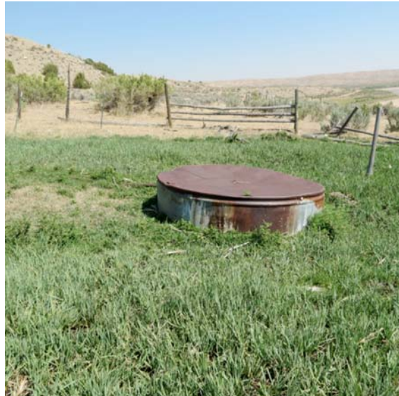
FIG. X1.11 Water Supply Well, Example 1
